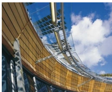
PV cells within glazed roof shading system
